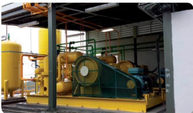
The equipment supply is completed with AP and BP feed pumps, continuous purging flash tank, purge cooling tank, steam silencers, field instrumentation, power panel and switchboards.
